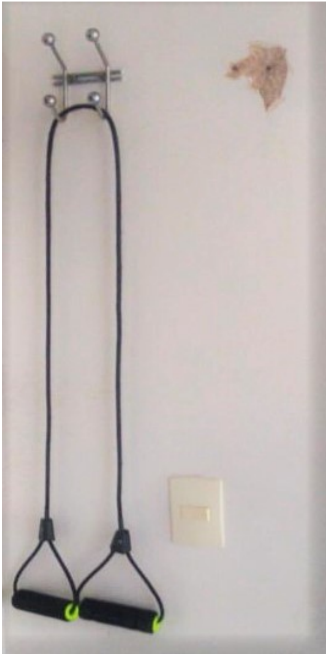
Figura 1: Elastic rubber band (ERB) used for working out and the detachment site of the wall hanger used as an anchor.
